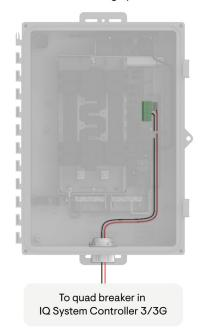
**NOTE:** The IQ Gateway L2 terminal is shorted to the L3 terminal using a jumper. While powering the L2 of the IQ Gateway, loosen the jumper from the L2 terminal, insert the wire, and then tighten it to ensure both the wire and jumper are properly installed. Do not loosen the jumper connection on the L3 terminal.
