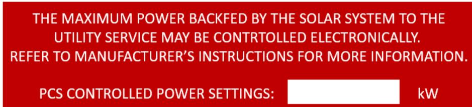
Recommended area to affix: On the dead front, below the transparent breaker, position the cover for the mains breaker.
